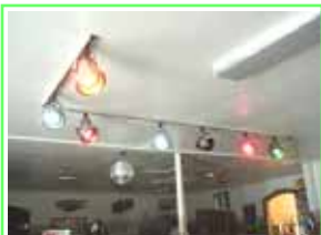
Ceiling Mounted Color Stage Lights (8)
