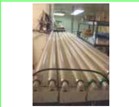
Lights, (6) 8ft. Shop , Double Bulb
