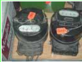
Electricity Meters, 2 "Westinghouse" c1930's
