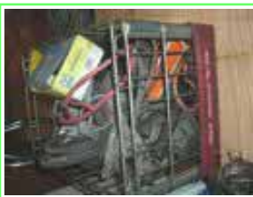
Parts & Wires in Metal Basket
